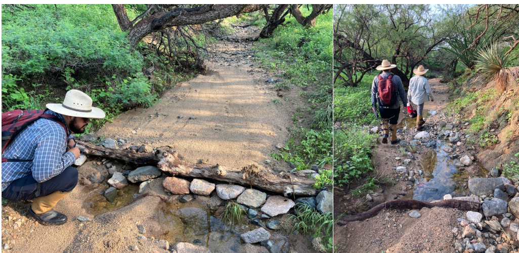
Figures 1 & 2. Erosion control structures, filled in with sediment after recent rains.
