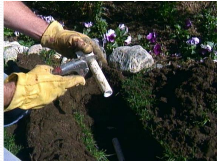
Repair of underground leak in irrigation line
