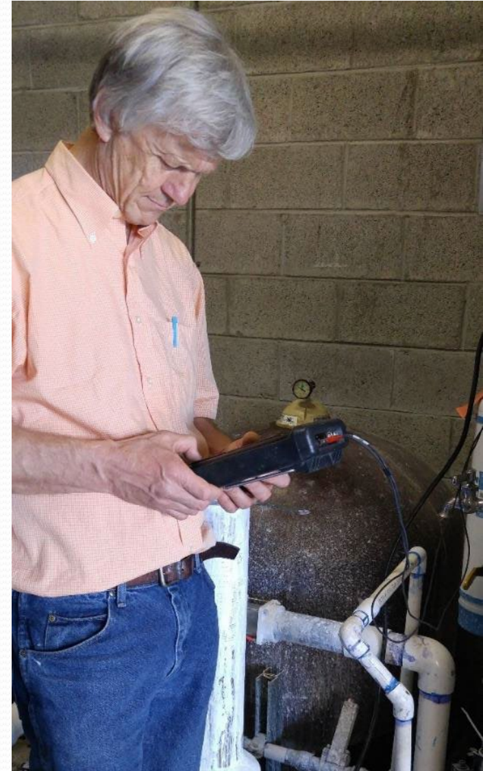
Deploying an ultrasonic flow meter at a pool to log unmetered flows
