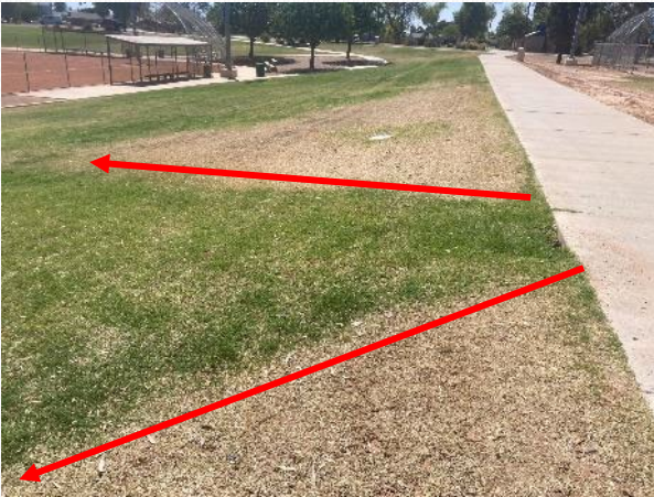
Missing irrigation head by sidewalk resulted in flood irrigation (note pattern of green grass)
