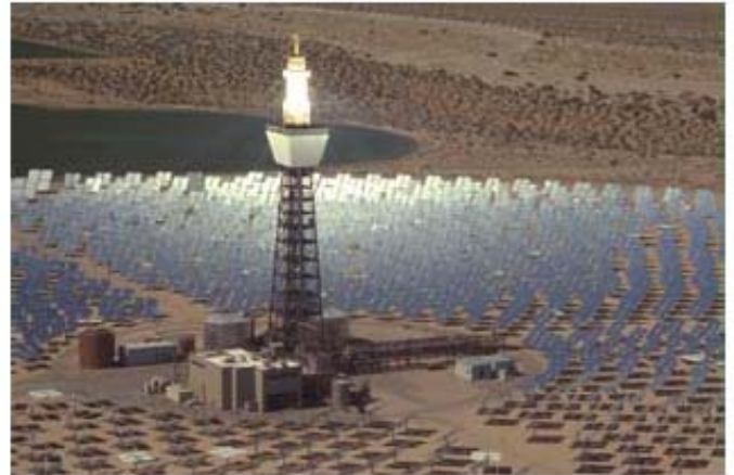
Figure 8: 10 MW power tower pilot project, Barstow, CA
