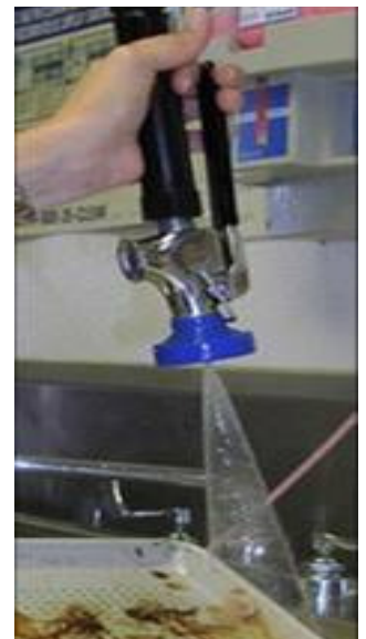
New 1.6 gallons per minute spray valves clean using greater velocity and lower water volumes.
